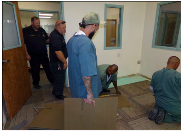
Newsroom construction [Photo courtesy of IR]
